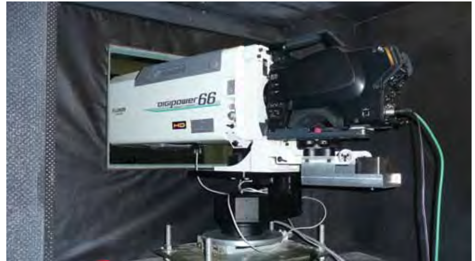
Magna Systems' installation of the new Camera Robotic Control Solution at Australia's Parliament House.
